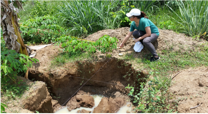
One of the tasks assigned to Sha is construction monitoring of the core house construction in Masagana Angat Resettlement Site. In this picture, she is taking measurements of the footing excavation to check if it is according to plan.
