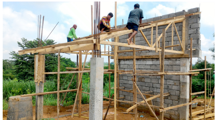
Top photo: Columns and firewalls have been constructed for the first batch of beneficiaries.
