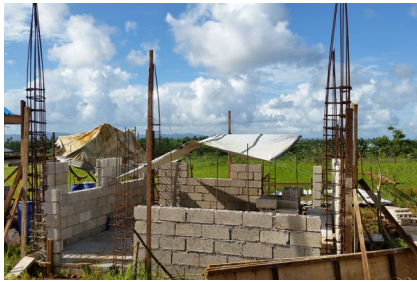
The Caga-ut single-detached house uses post and lintel construction system with walls made of concrete hollow blocks.
