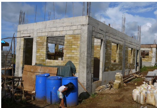
Two duplex houses have walls made of interlocking compressed earth blocks.
