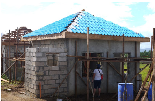
Micro concrete roof tiles have been laid out for this single-detached house.
