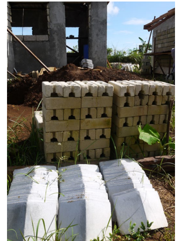
Alternative building materials such as micro concrete roof (MCR) tiles and interlocking compressed earth blocks (ICEB) were used for the Caga-ut Shelter Project.
