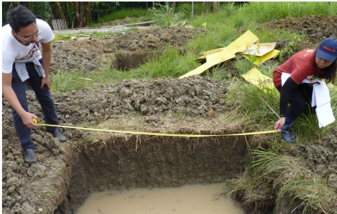
Niña (right) together with her fellow UST intern Erol Enriquez measures the footing excavation made for the housing project of Masagana Angat.
